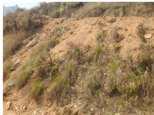
Figures 6 a, b, c, and d: Photographs of overburden at site during taken 2024 site visit showing unstable slope and debris
